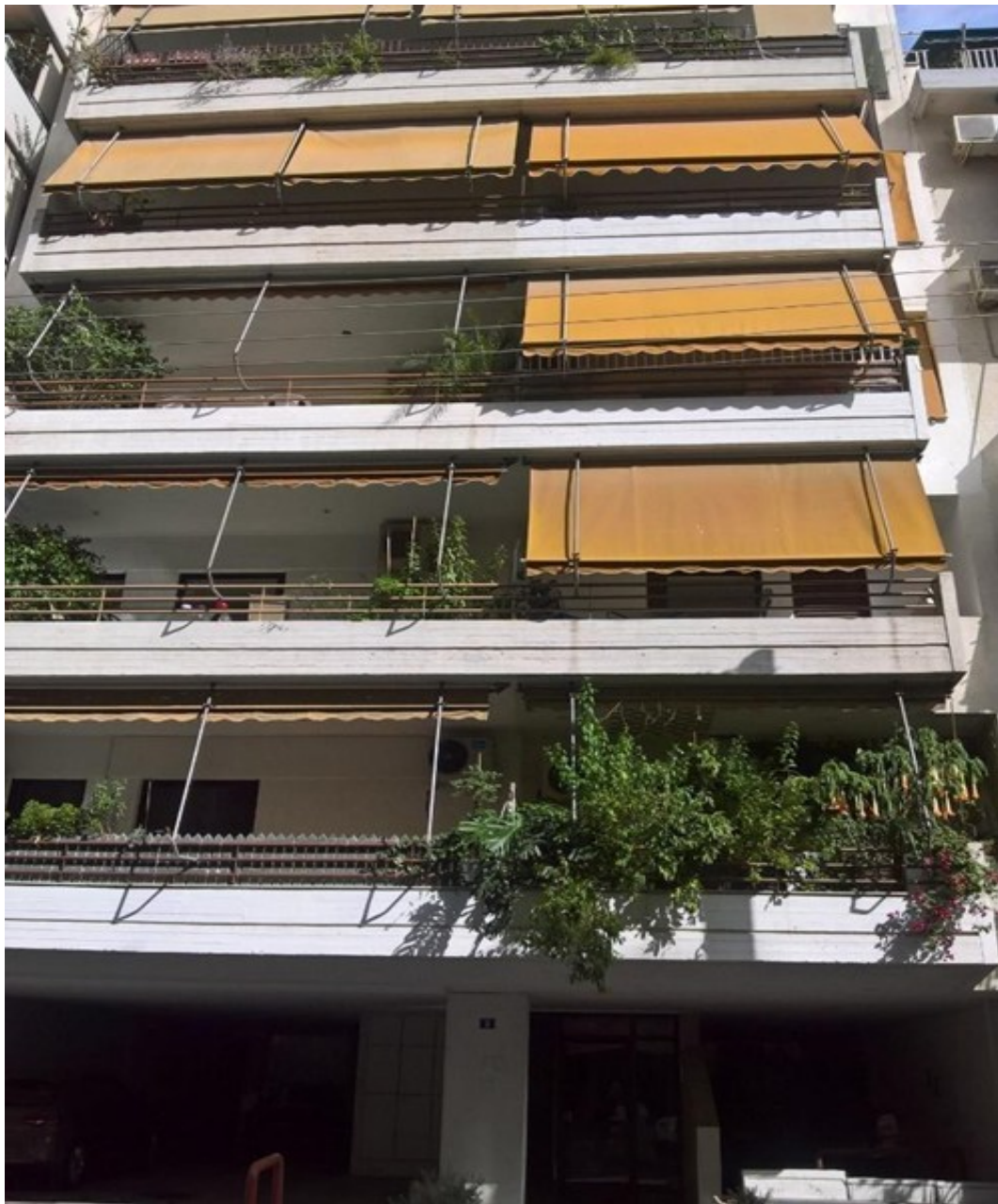
Figure 9. The front view of the apartment building. The main use on the ground floor is parking space. Source: Personal archive
